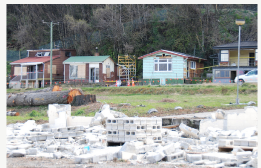
Salvaged bricks at Lakeview Deconstruction, QLDC.
