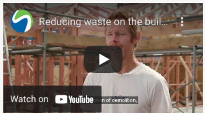
Hamilton example of onsite waste minimisation
