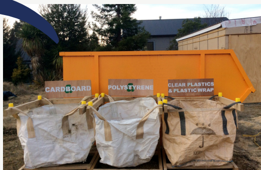
Example of an onsite recycling segregation station by Dunlop Builders.
